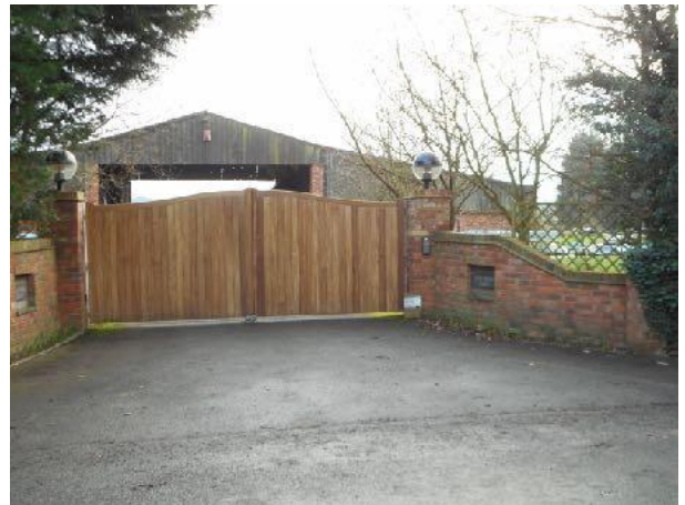
Fig 96 Five Oaks Farm entrance
